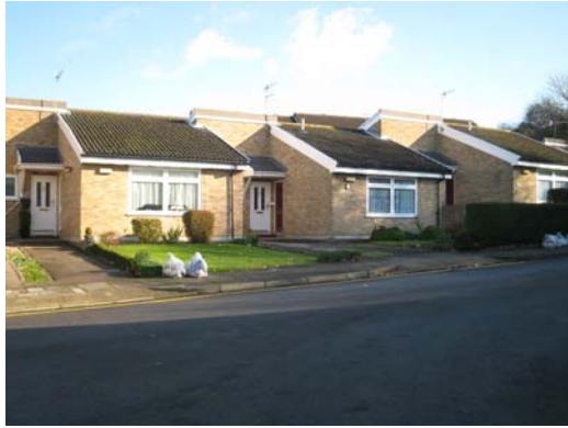
(example of a bungalow at Brymore road)
